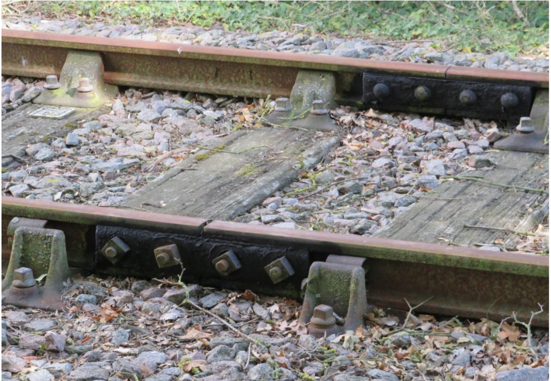
Figure 6 Rail joint near Knodishall in ambient temperature of 18°C
